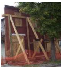
Stabilizing vacant buildings
